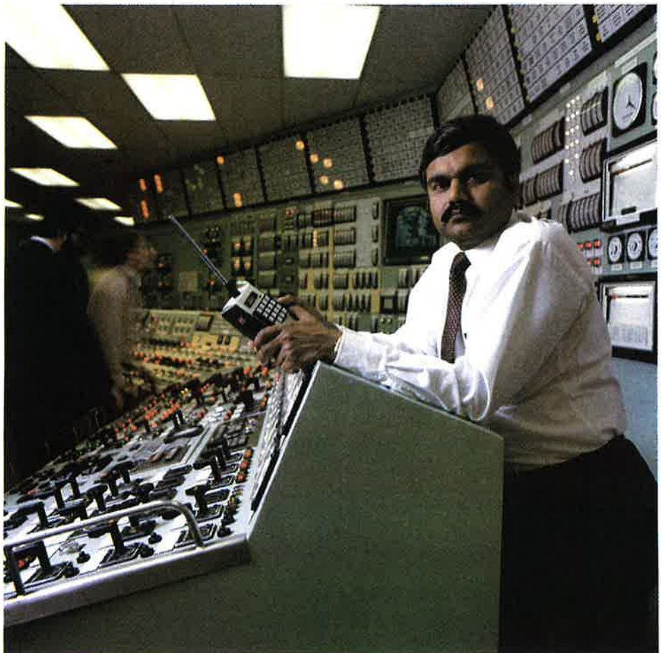
Arvind Patel in control room at North Anna nuclear power plant. It's not the real control room, however. It's the simulator he built to train those who operate the real one.
